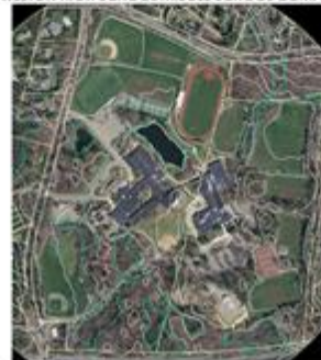
FACILITY INSPECTIONS + OBSERVATIONS
