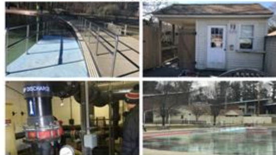
FACILITY INSPECTIONS + OBSERVATIONS
