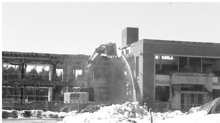
*Demolition of the old Field School was delayed due to a change in the state regulations for the removal of hazardous materials. Additional asbestos was discovered in mastic found under the base of walls*
